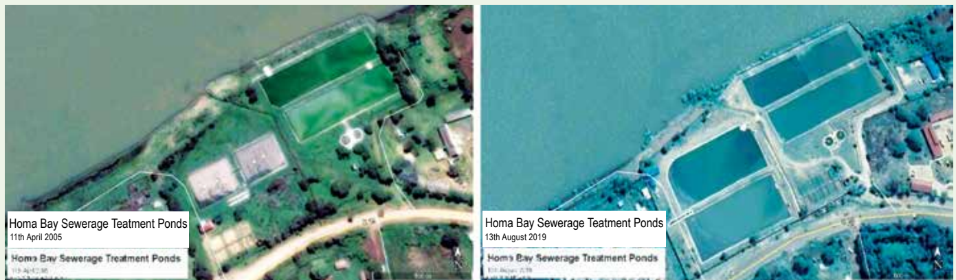
Figure 41: Google Earth Image extract of Homa Bay Sewerage treatment ponds showing poor siting of the ponds and the extent of submergence of from Lake Victoria level rise lading to direct contamination of Lake waters
