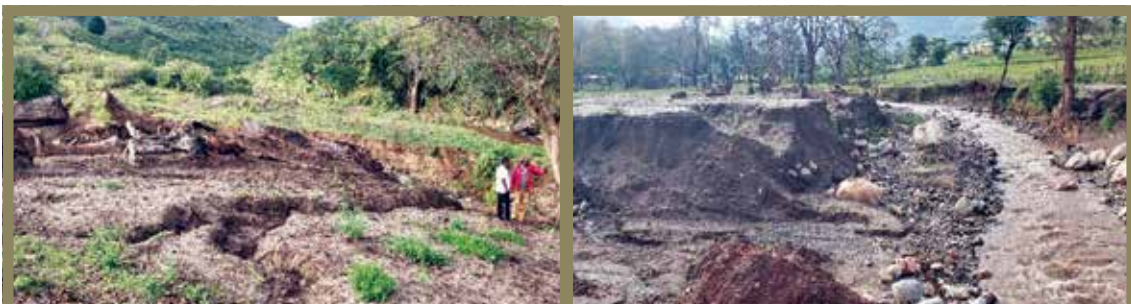
Plate 7: Evidence of landslide hazard at Sebit Bridge at the confluence with Muruny River and at the Sebit stream.
