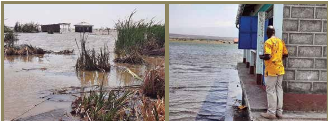
Plate 6: Evidence of flood impacts from the rising water levels in the lakes affecting infrastructures as far north as Ileret (Left business facility) and South as Loinyangalani (right refrigeration house) both in Marsabit.
