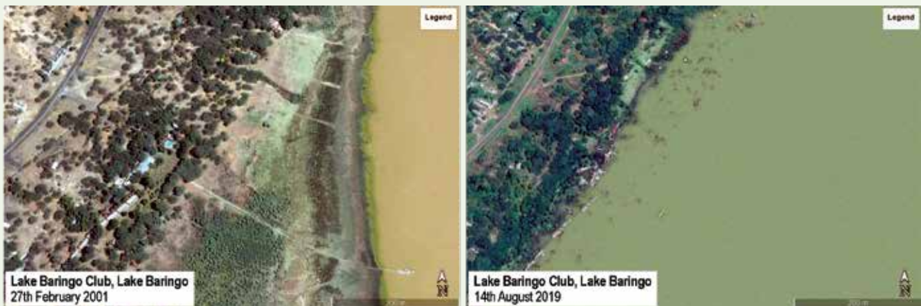
Figure 33: Evidence of the extent of flooding from the rising lake Baringo level and the damage it has brought to the development infrastructure (from Google Earth images of Feb 2001 and August 2019)
